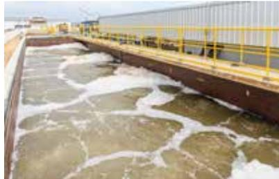
This is the heart of secondary treatment. Microorganisms like bacteria and protozoa consume and break down the organic matter left in the wastewater after primary treatment. While there are different types of biological treatment systems, all utilize these hardworking microbes.
