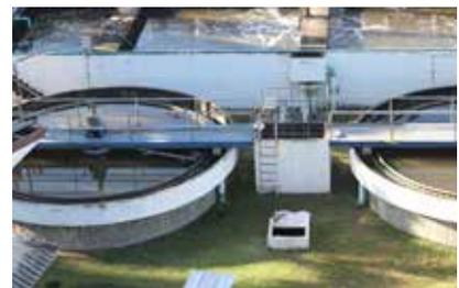
Heavier organic matter sinks to the bottom as sludge, while lighter materials like oils and fats float to the surface and are skimmed off.
