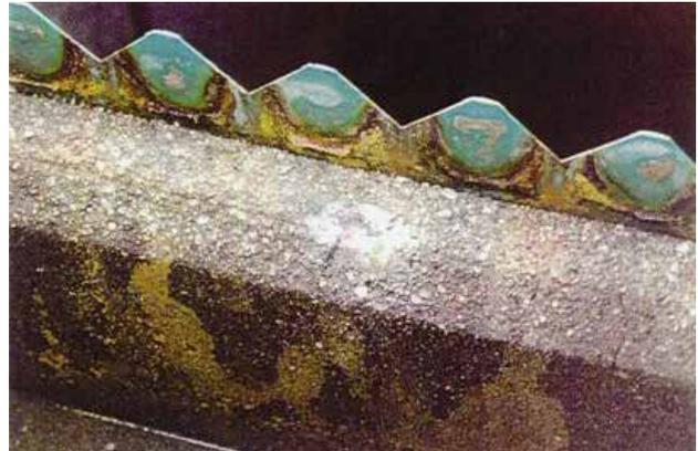
acid attack (BSA) or microbial induced corrosion (MIC) is usually the most serious cause of damage in covered areas where there is turbulent sewage. Sulfuric acid can cause concrete erosion rates of 0.5 – 10.00 mm per annum; in extreme cases erosion of up to 20 mm has been measured.
