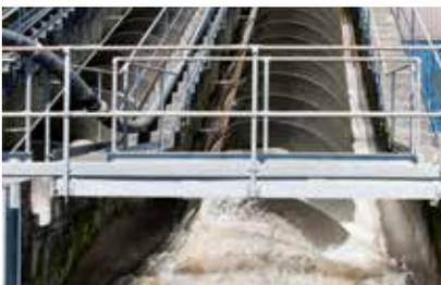
This stage removes large objects like rags, plastics, and debris that could damage equipment later in the process.
