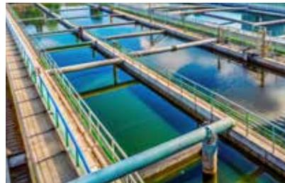
While primary disinfection often occurs after secondary treatment, some facilities may add another disinfection step, using processes like chlorine or ultraviolet light, to ensure even stricter removal of bacteria.
