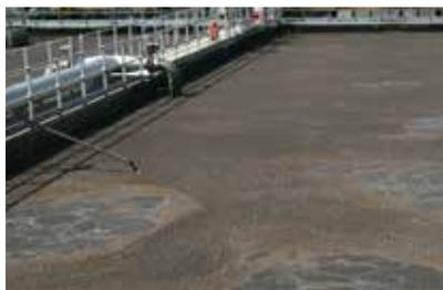
Next, the water flows through a grit chamber where heavy, inorganic materials like sand and gravel settle out.
