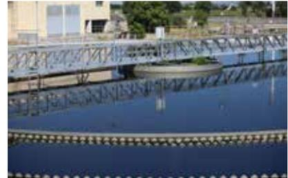
After the biological breakdown, the water enters a settling tank again, allowing the microorganisms and any remaining solids to separate from the treated wastewater. It's like letting the water settle after the microscopic cleaning bacteria have done their job.
