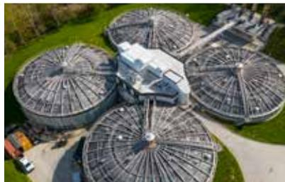
Sealed vessels allow organic waste break down through a process called anaerobic digestion. Microorganisms, like bacteria, break down the waste in an oxygen-free environment, producing biogas (mainly methane) as a byproduct.
