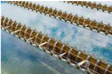
Treated water may pass through filters, such as sand filters or membrane filters, to remove any remaining particles.
