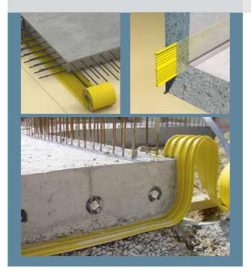
PVC profile waterstops for joint sealing
