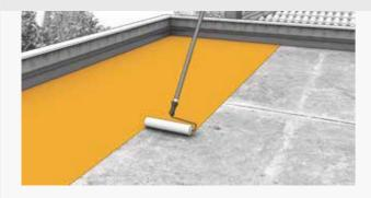
Rubberised bituminous waterproofing coatin
