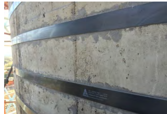
Contractor : Teichmann Structures
