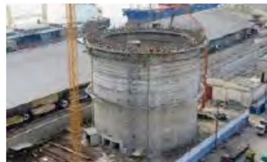
Owner: CIM IVOIRE Controller: INTERCEM Project Manager: IC CONTRACTOR
