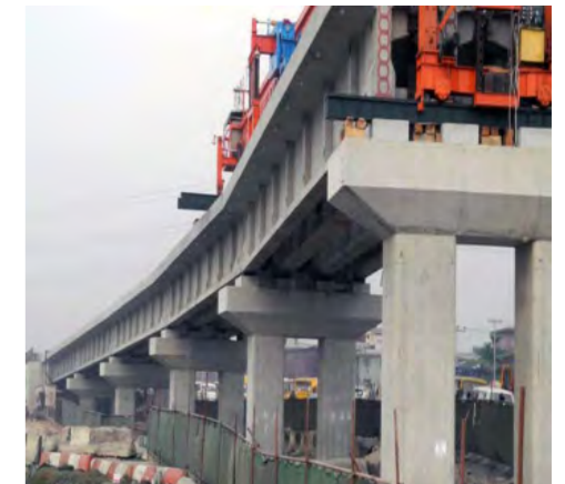
Owner: Lagos Metropolitan Area Transport Authority (LAMATA) Contractor: China Civil Engineering Construction Corporation (CCECC)
